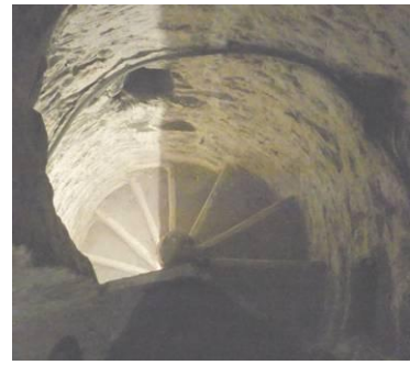
Figure 1 Stairs inside the tower
